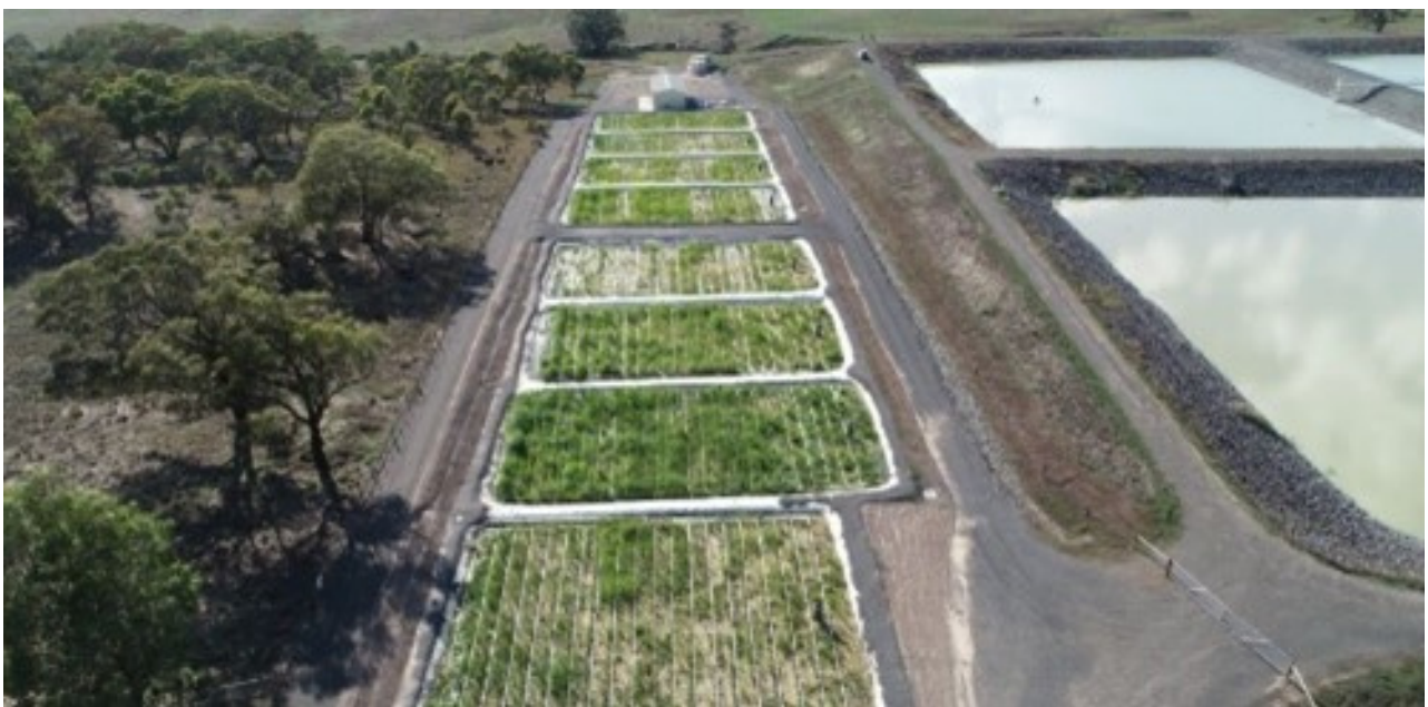
Kilmore (Vic): Goulburn Valley Water met nutrient discharge requirements at lower cost, improved the health of a degraded waterway, and saved greenhouse gas emissions by fencing stock out of waterways, riparian plantings and erosion rehabilitation.
