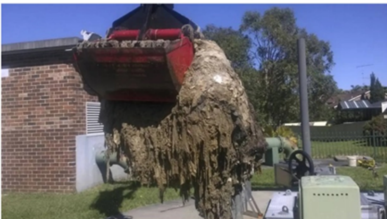
Sydney Water workers at the Shellharbour sewage pumping station cleaning out a blockage of wet wipes. A spokesman said such clean-outs happen on a regular basis. ILLAHARISA PERELBY
