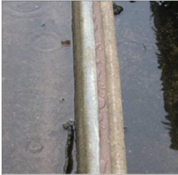
Figure E-3: FRP Cover Sections Sealed with flexible, air tight sealant. This image is taken from a wastewater treatment plant odour cover and shows a flexible sealant (e.g an appropriately UV stable and corrosion resistant SikaTank) sealing the join between two odour covers
