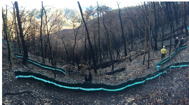
Sediment fences installed in high-risk bushfire affected headwaters (Gary Sheridan, The University of Melbourne).
