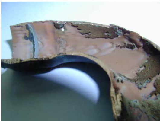
Typical erosion-corrosion of copper pipe
