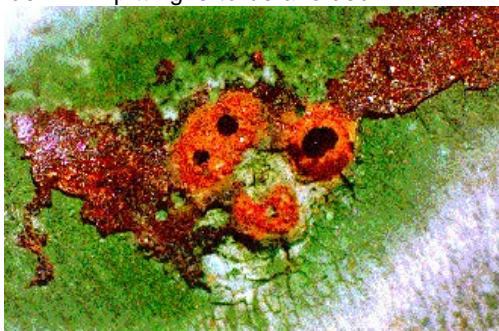
Internal pitting of copper pipe surface
