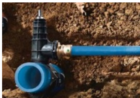
FIGURE 4 GEOPRESS K TAPPING VALVE
