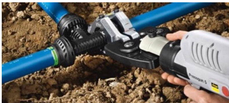
FIGURE 1 PRESS JOINT
