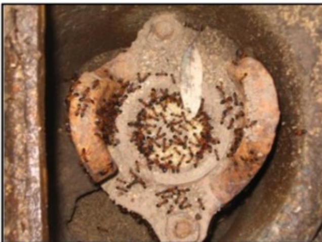
Figure 3: Ants infested hydrant with reappearance of ants 3 weeks after cleaning
