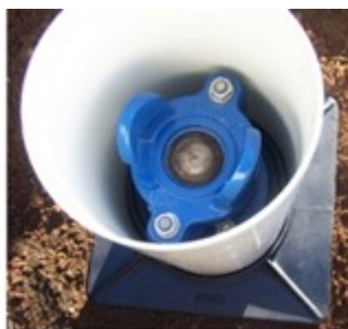
FIGURE 2 SHROUD PIPE INSTALLED
