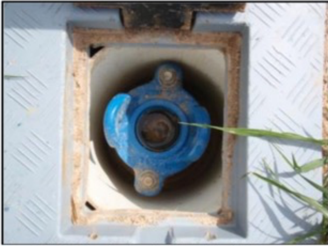
Figure 4: Hydrant head replaced and installed with hydraguard boot (March 2011)
