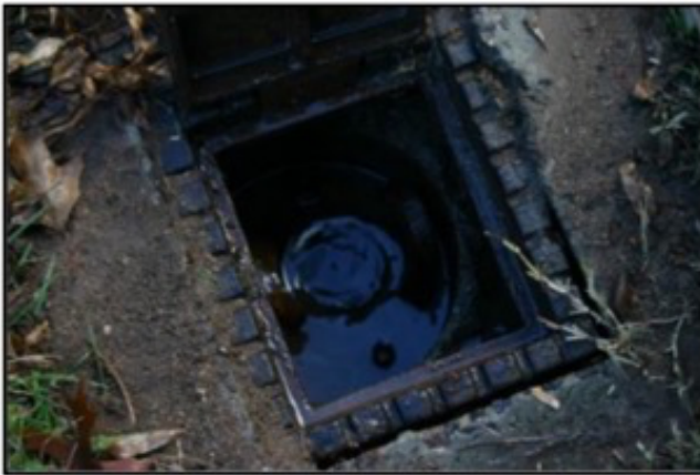
Figure 2: Ants infested hydrant after being cleaned with high pressure hydro digger
